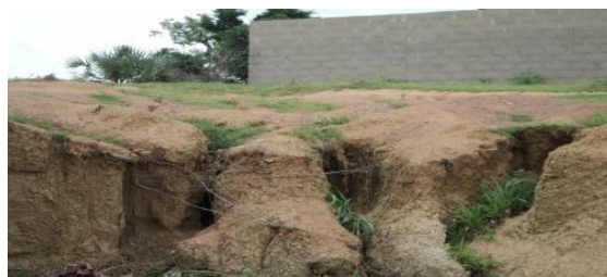
Figure 2f: Gully erosion site at Sangere-MAU
