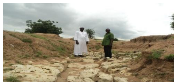
Figure 2j: Gully erosion site at DagriWuro Alhaji
