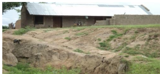
Figure 2g: Gully erosion site at Vunoklang
